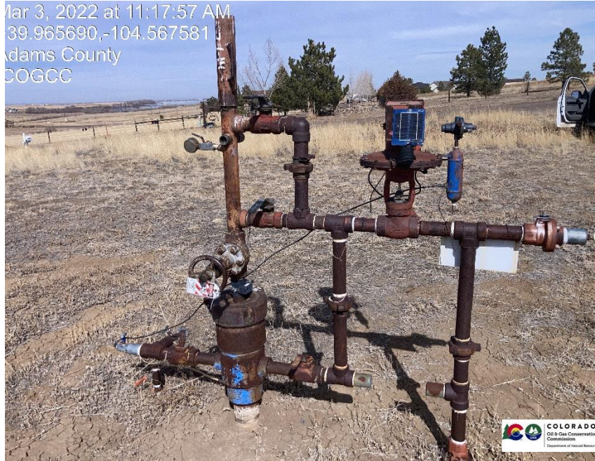
Pic 3 wellhead, master valve and flowline valves were in the close position at time of inspection.
