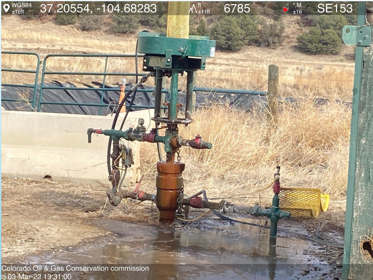
PHOTO 4: PACKING ON WELLHEAD IS LEAKING. REPAIR LEAK CA DATE 3-4-2022.
