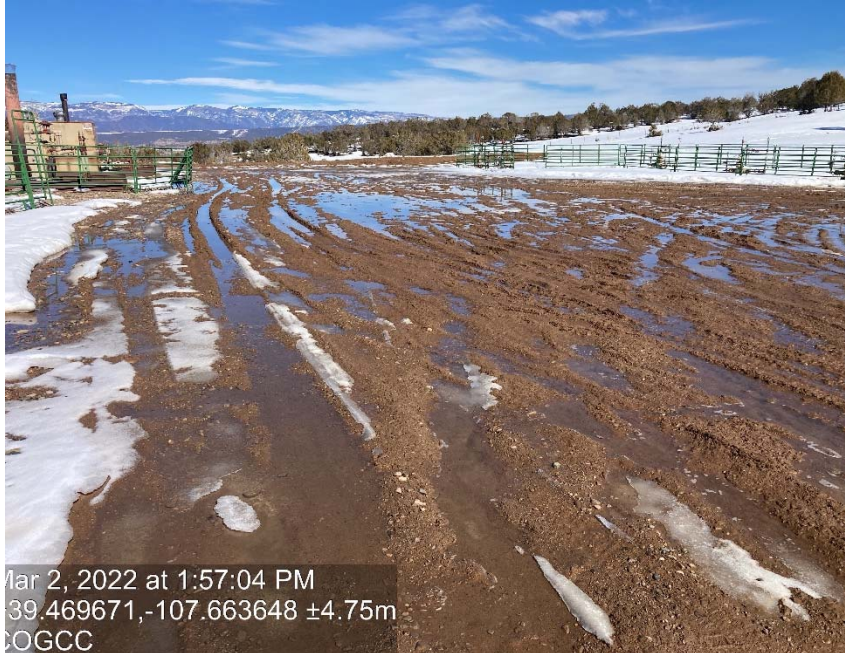
Lack of stabilization/compaction
