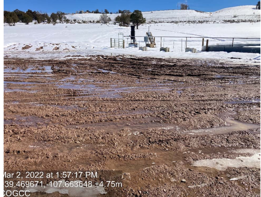
Lack of stabilization/compaction
