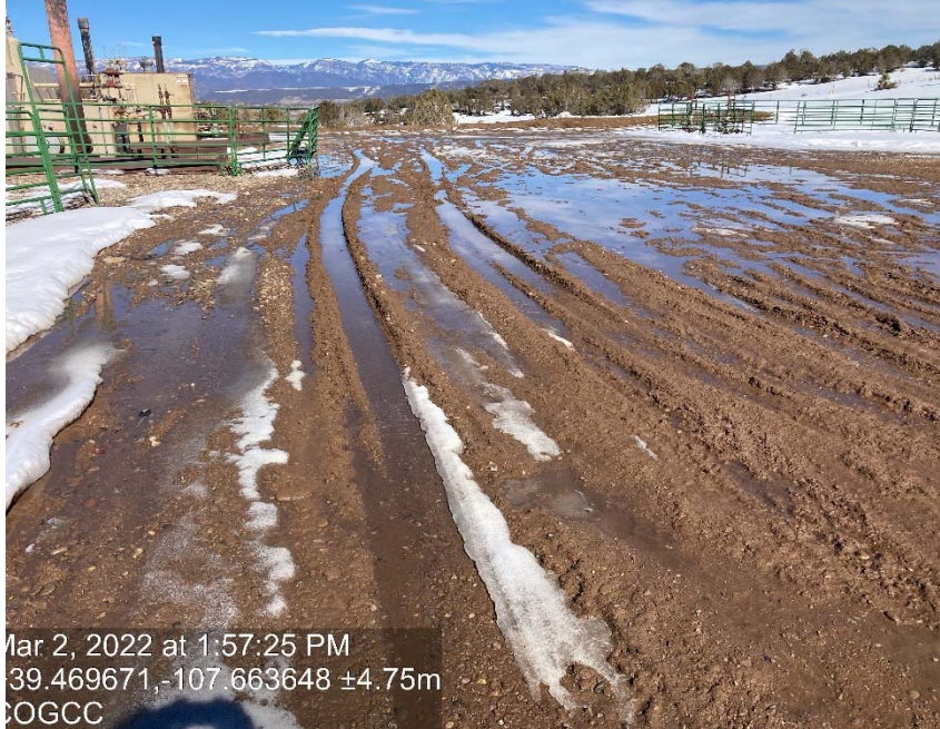
Lack of stabilization/compaction
