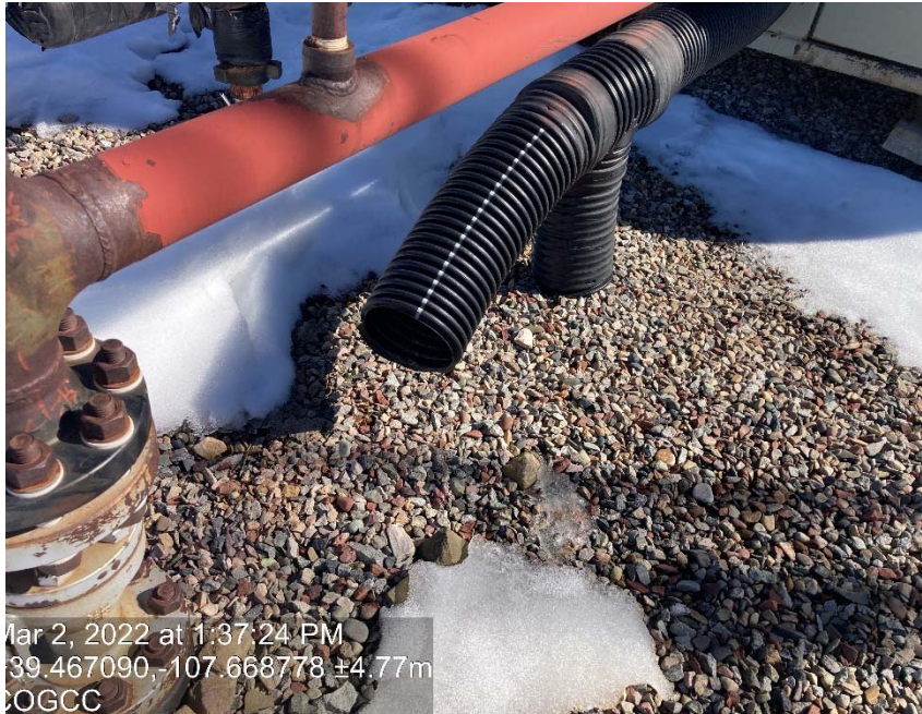
Open exhaust thaw lines
