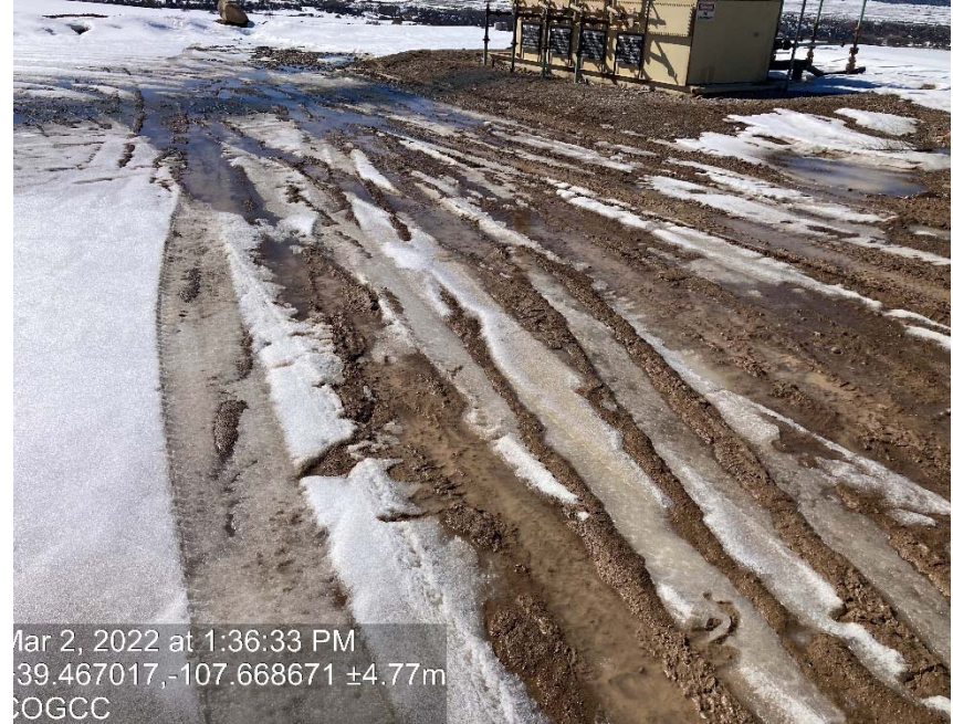
Lack of stabilization/compaction
