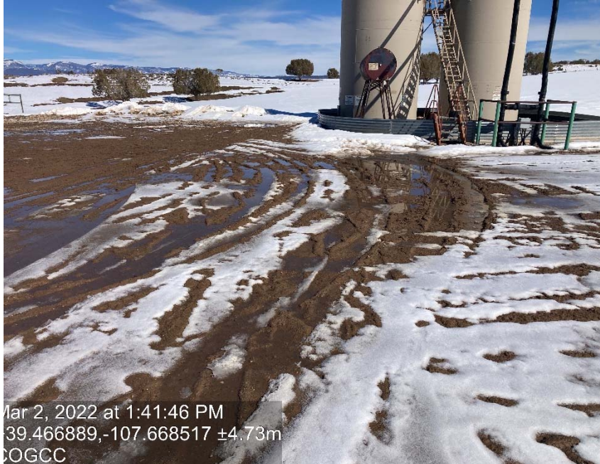
Lack of stabilization/compaction
