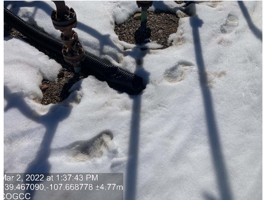
Open exhaust thaw lines
