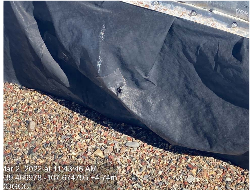
Holes in containment
