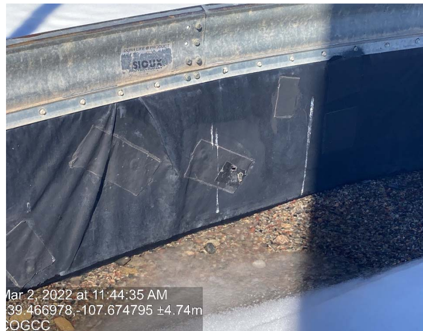
Holes in containment
