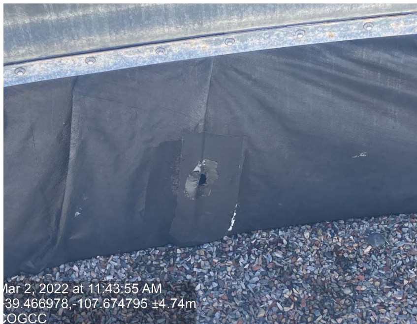
Holes in containment
