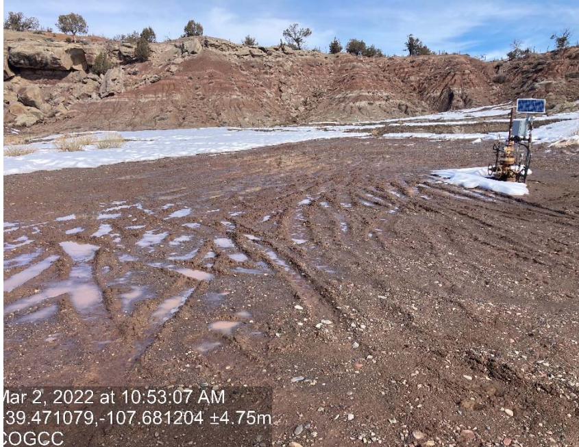
Lack of stabilization/compaction
