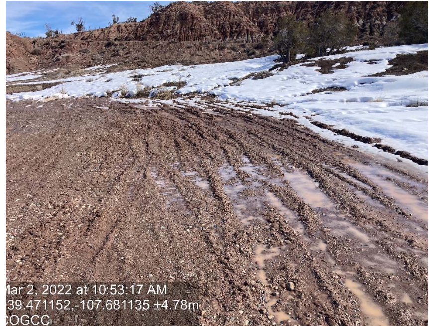
Lack of stabilization/compaction
