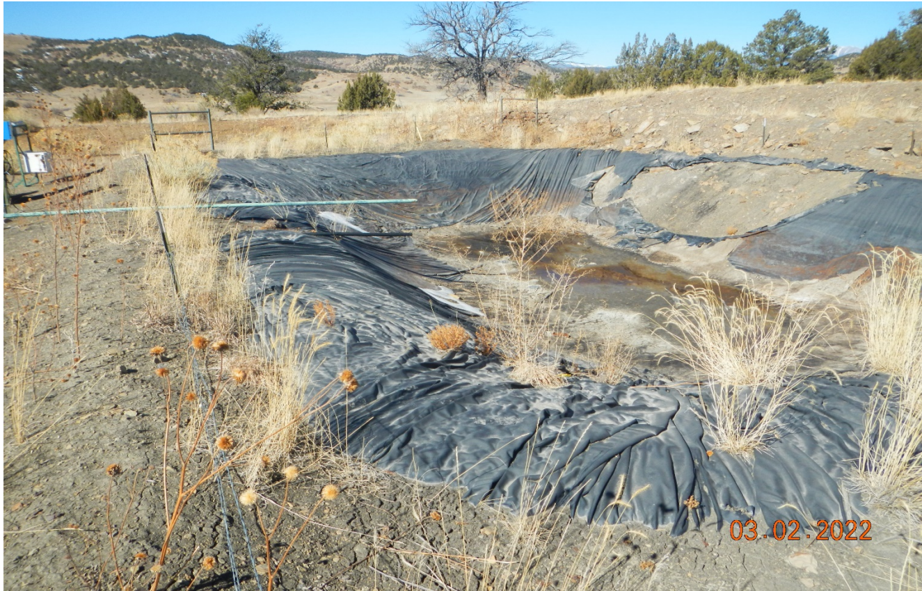
Photo 3. Facing toward the pit. The pit liner is torn and degraded. The fence around the pit is not maintained.
