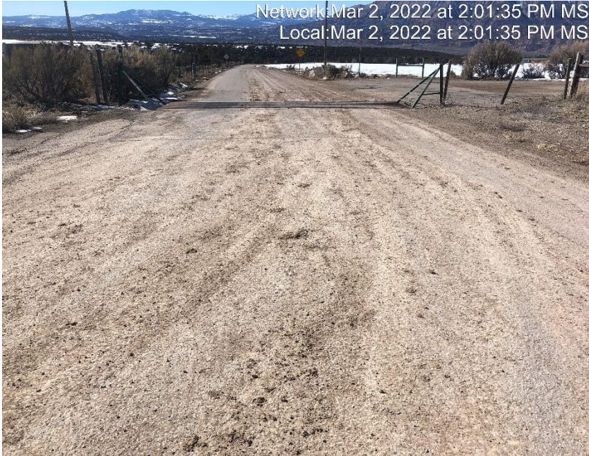
Photo #6074 Sediment has been transported on to County road 306 for approximately 100 yards.
