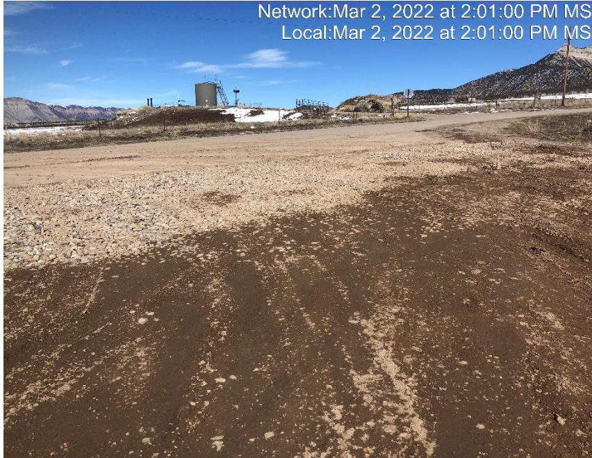
Photo #6072 Insufficient tracking BMP at entrance to location
