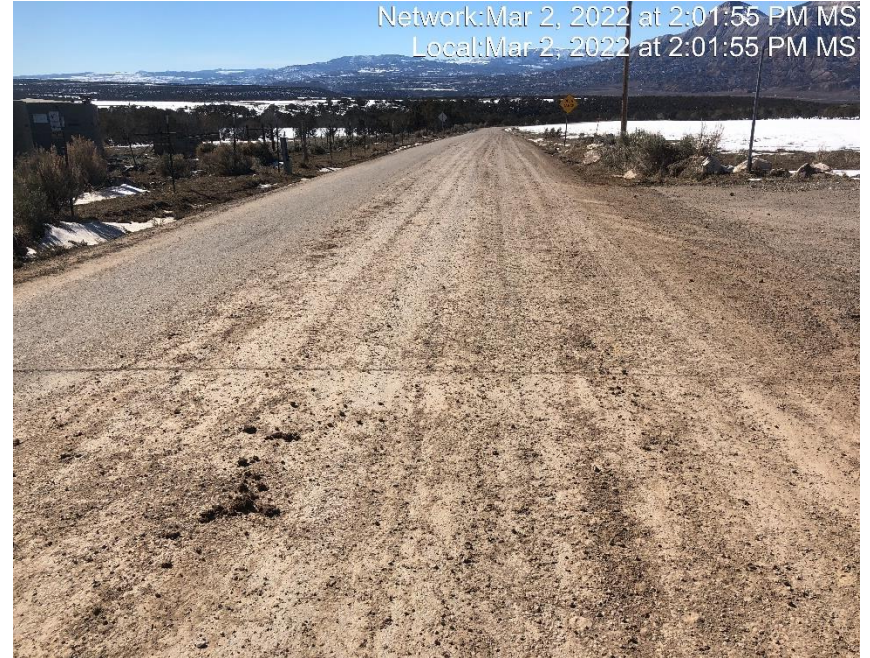
Photo #6075 Sediment has been transported on to County road 306 for approximately 100 yards.
