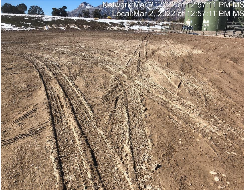
Photo #6065 Location lacks stabilization.
