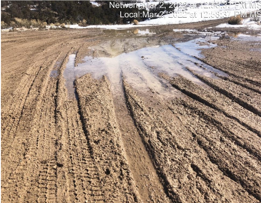
Photo #6067 Insufficient tracking BMP at entrance to location.
