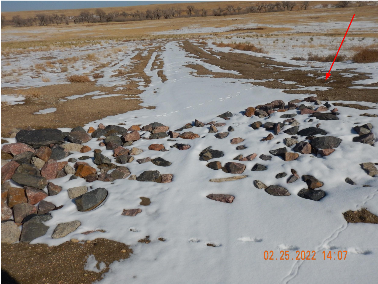
Photo 2. Photo taken from the eastern tank battery, facing East. Photo illustrates Operator has performed additional stormwater repair work but has not seeded the area. Some rill erosion was observed (red arrow) and should be repaired when performing seedbed prep.
