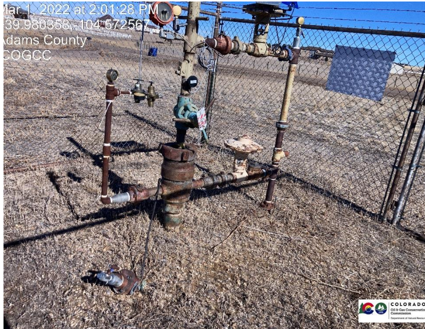
Pic 1 Penny 32-8 Master valve is in the closed position, all ball valves on flowlines, and casing are in close position. Bradenhead valve is in closed position.
