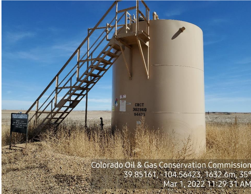
Photo 3: Tank Battery Sign
