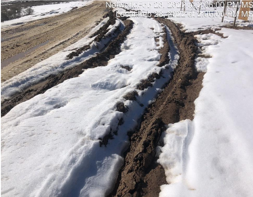
Photo #6050 Location lacks stabilization.
