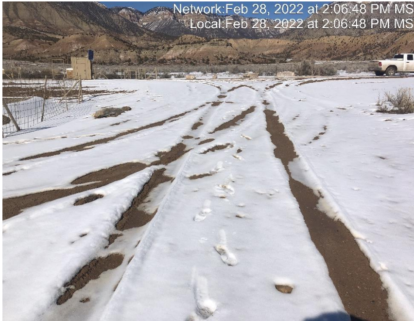
Photo #6052 Insufficient tracking controls at entrance to location.
