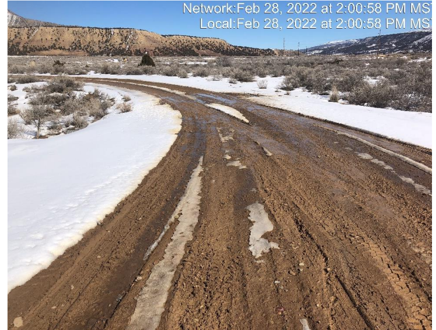
Photo #6047 Insufficient tacking control at entrance to location.
