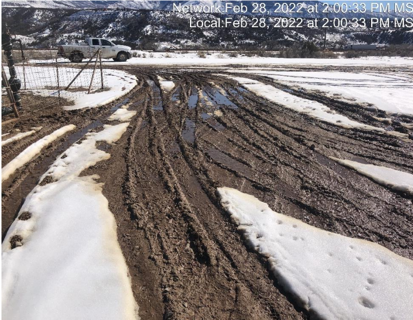
Photo #6046 Location lacks stabilization.
