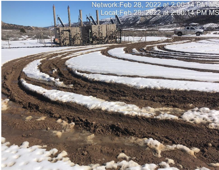
Photo #6045 Location lacks stabilization.
