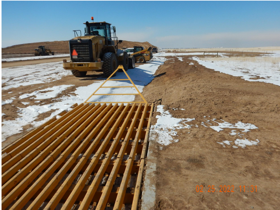
Photo 2. Photo taken from the entrance of location, facing West. Photo illustrates a ditch BMP that has been installed around the entire perimeter of location, which is directed to a stabilized outlet. Culverts are in process of being installed.
