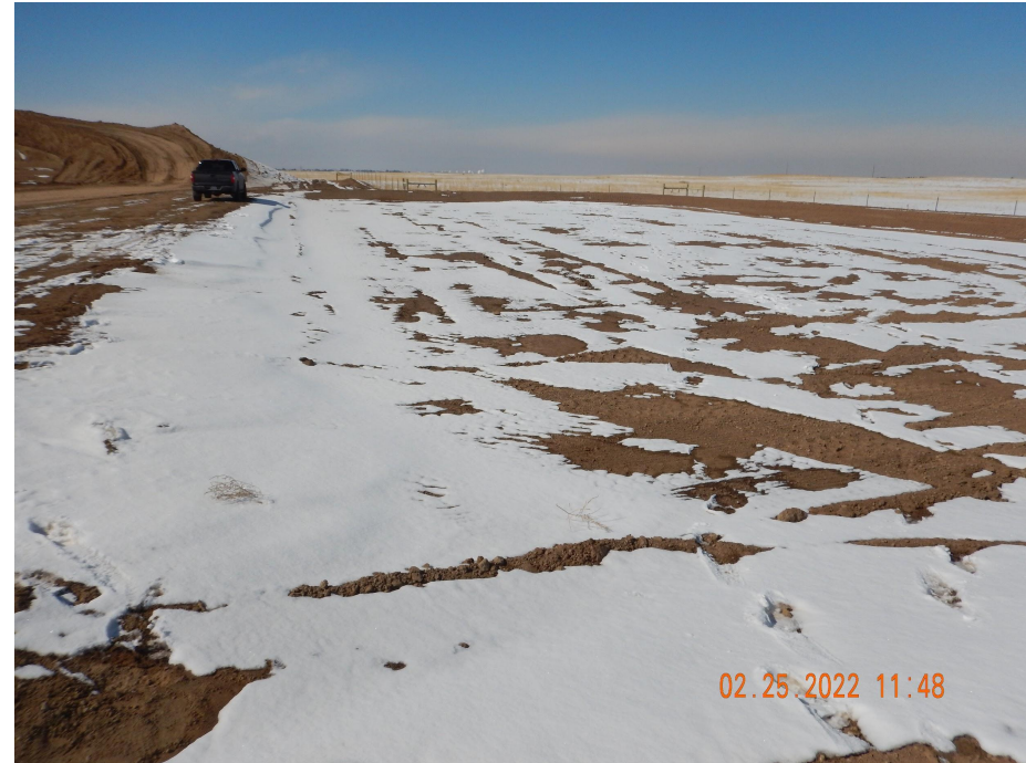
Photo 7. Photo taken from the northwestern location, facing West. Photo illustrates the sediment basin that has been engineered for a one hour, 100-year storm event.
