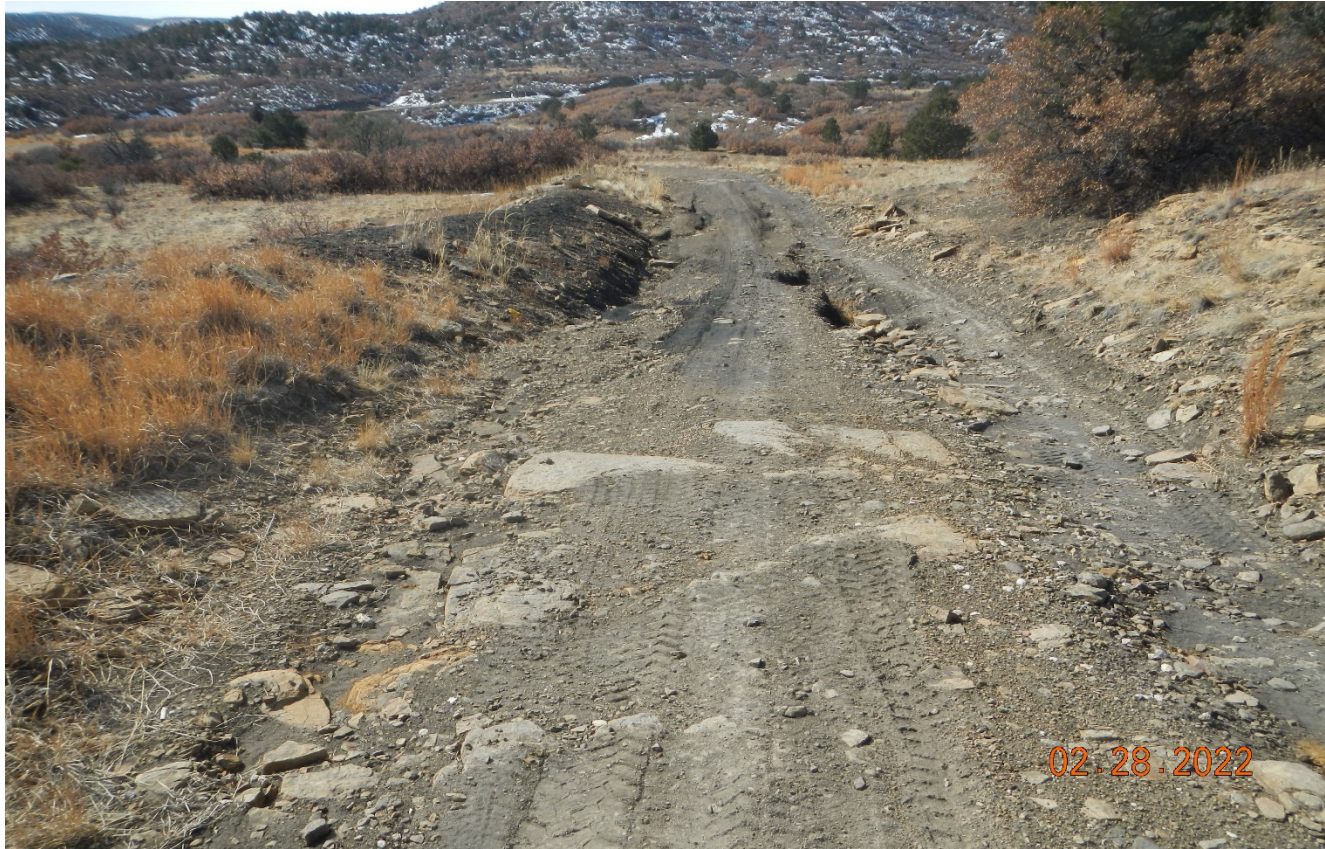
Photo 3. Facing south along the access road. There is erosion along the road that needs to be repaired and stabilized. This area has not yet been repaired
