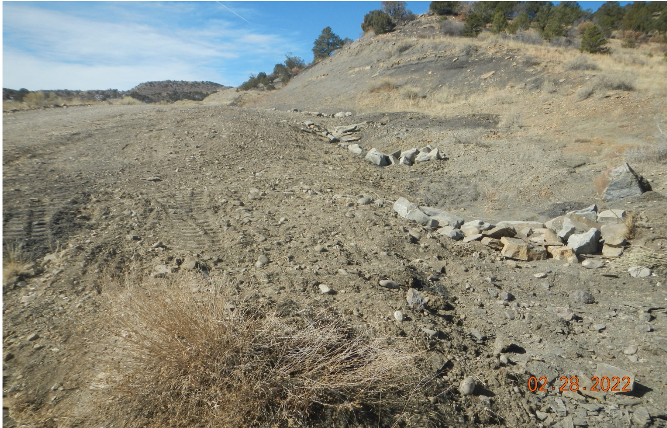
Photo 2. Facing southwest along the main road to the well site. There area rock check dams installed along the road side and areas of erosion have been repaired.
