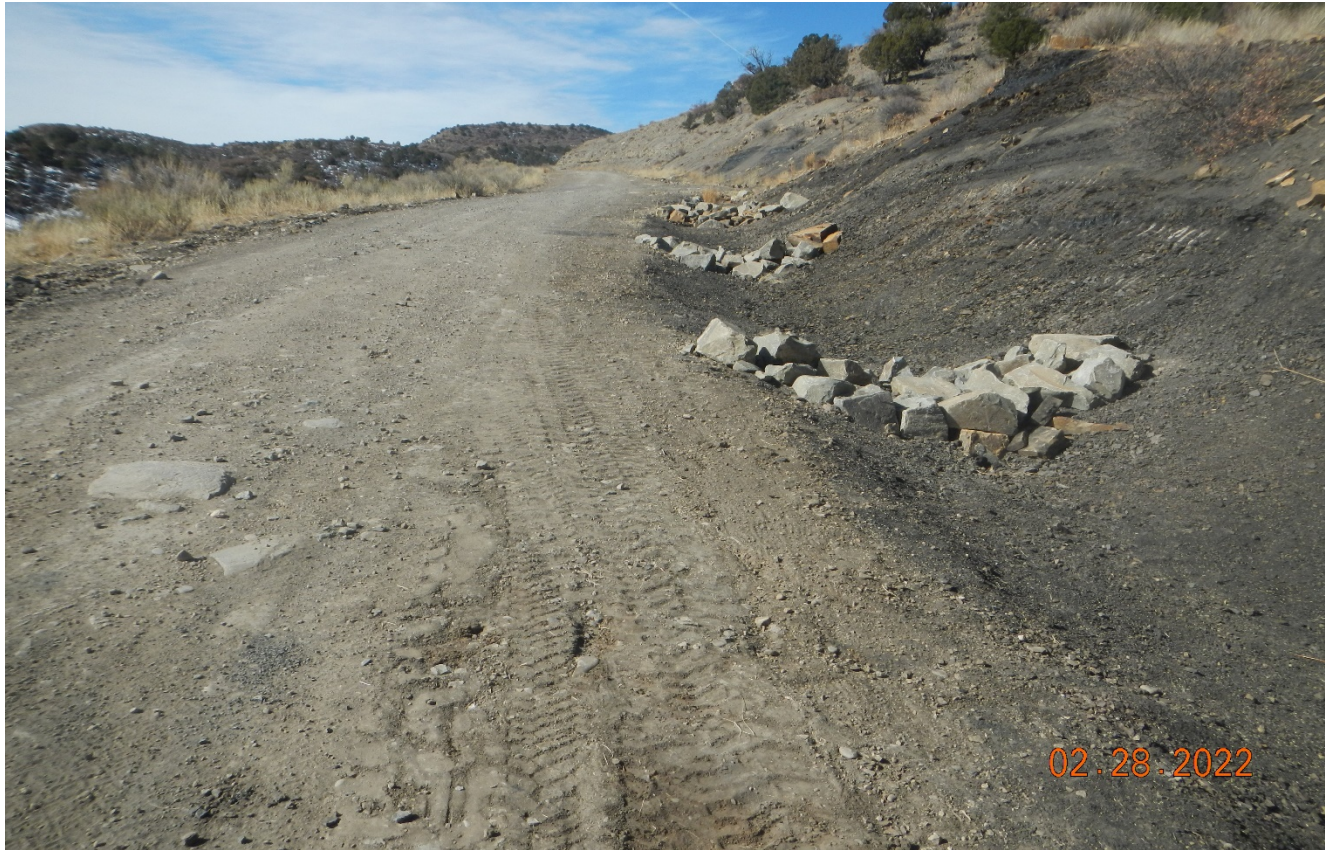
Photo 3. Facing southwest along the main road to the well site. There area rock check dams installed along the road side and areas of erosion have been repaired.
