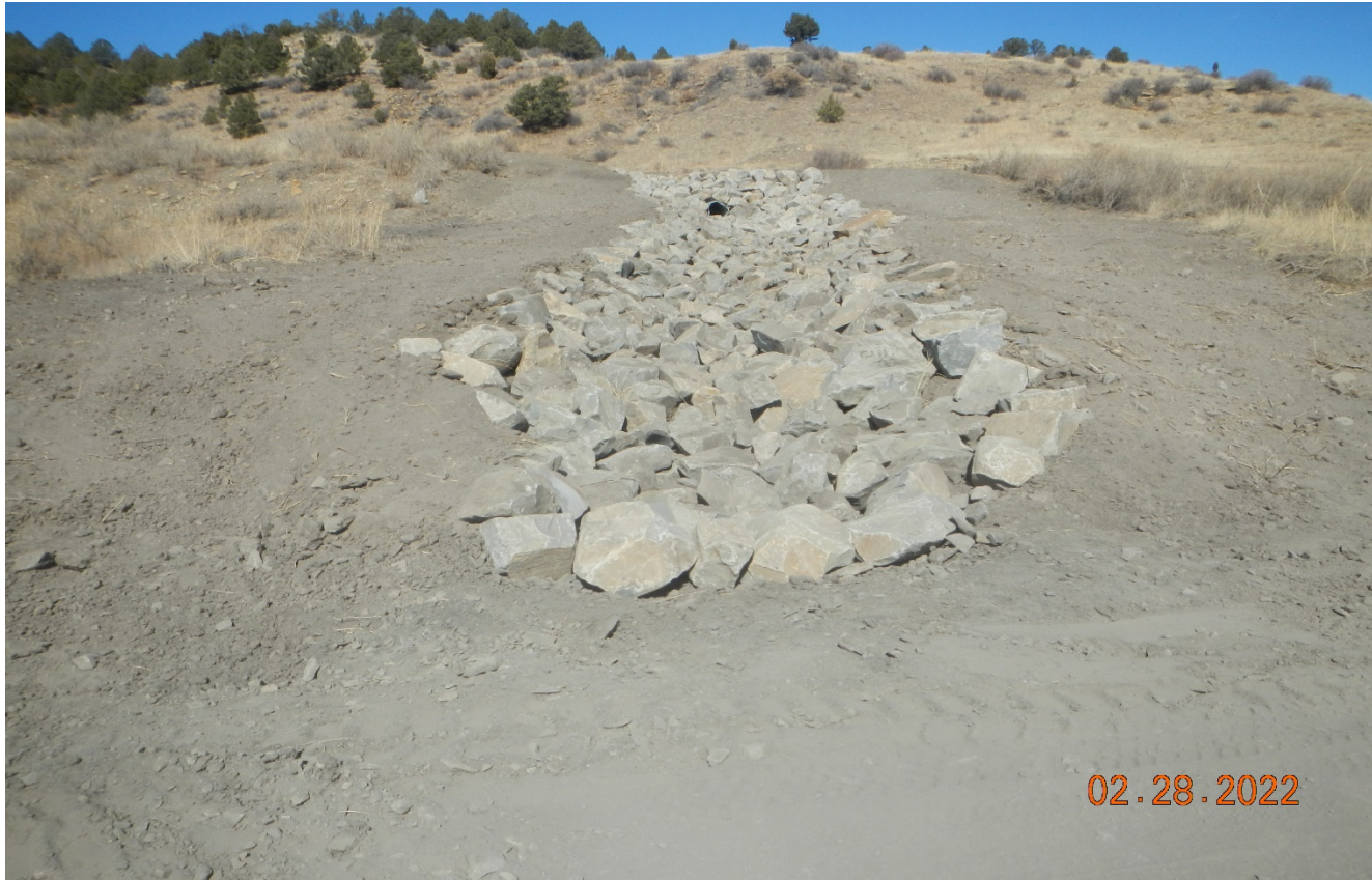
Photo 1. There has been rock rip/rap outlet protection installed at the culvert near the main road in Lorencito Canyon. Disturbed areas have been seeded.
