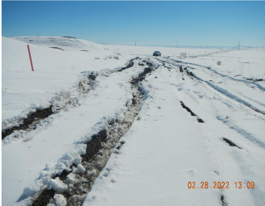
Location lacks compaction/stability
