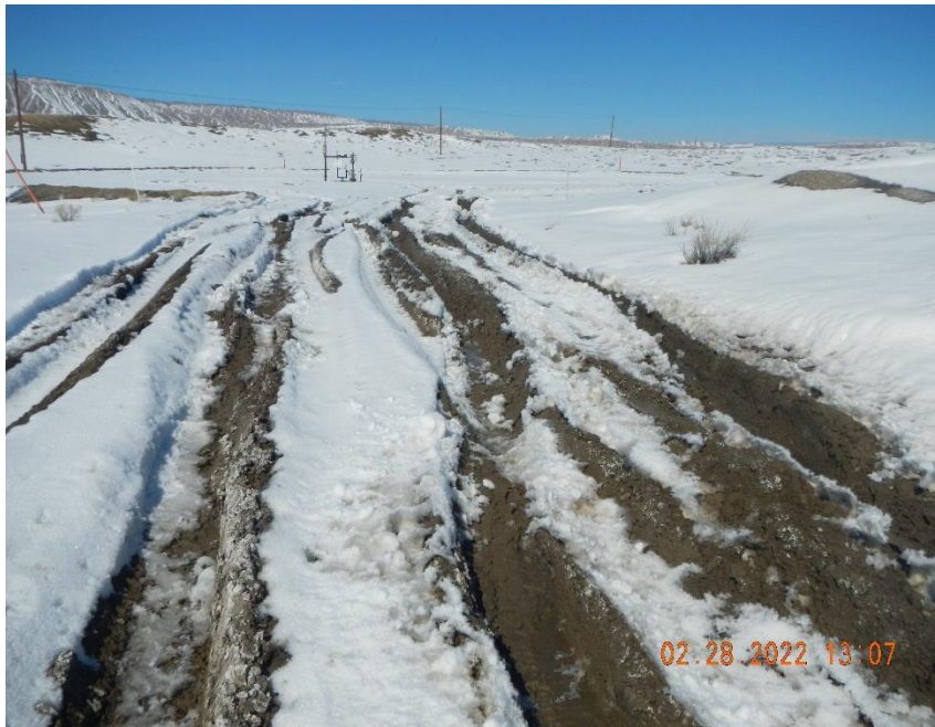
Access road lacks compaction/stability
