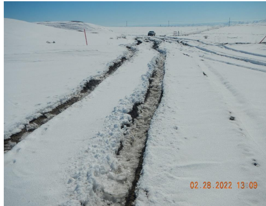
Location lacks compaction/stability
