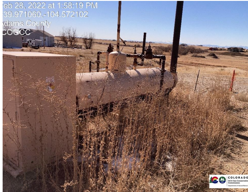
Pic 3 Separator, and abandoned midstream.
