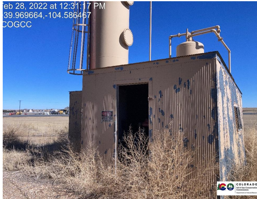
Pic 3 verticle separators, 1 heated. Unable to access separator house due to condition of building
