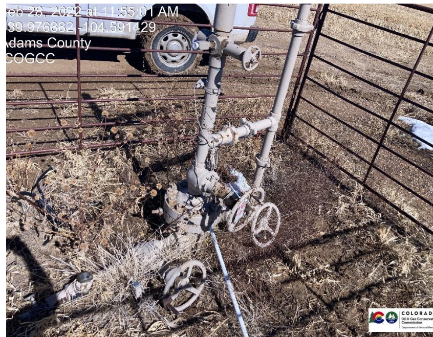
Pic 2 wellhead after LOTO, master valve is seized in position, appears open, but sales line appears to be shut. Casing valves are in close position,
