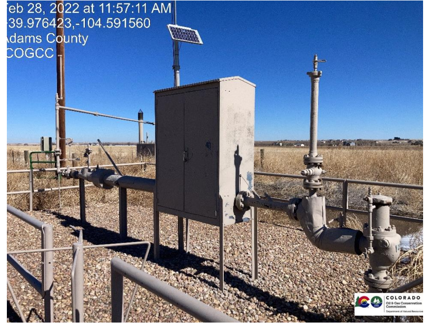
Pic 4 gas meter run
