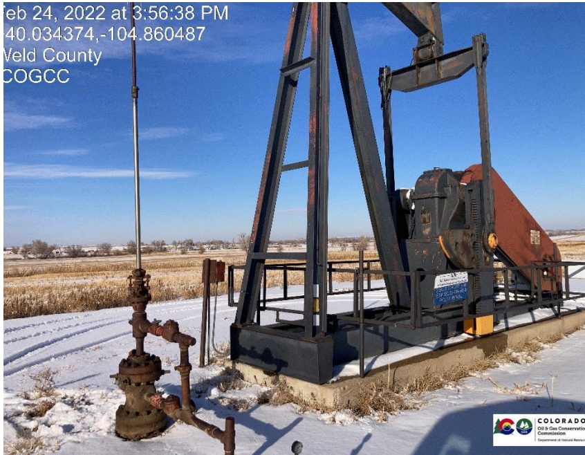
Pic 1 wellhead / pumpjack, electric equipment
