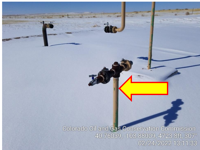
Photo 5 – Unmarked Riser
