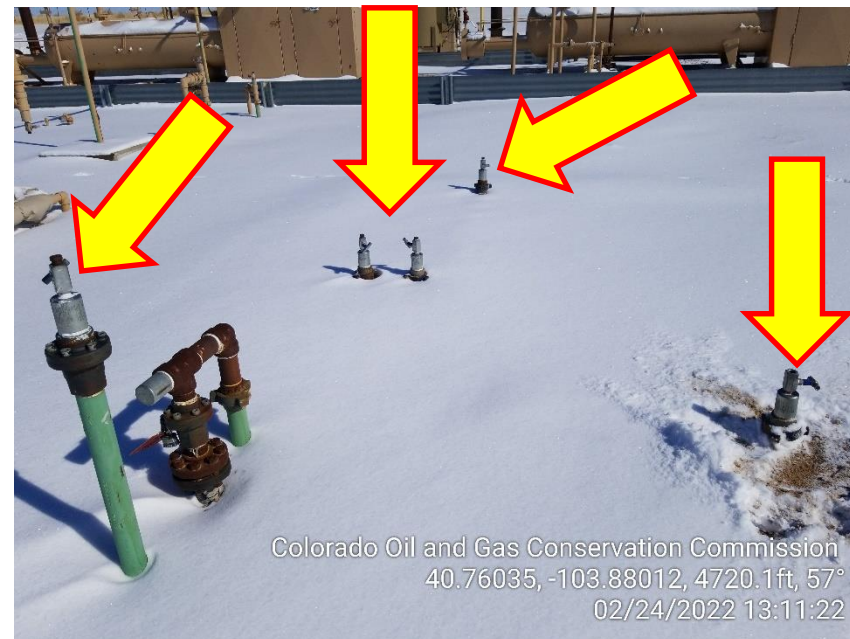
Photo 4 – Unmarked Risers
