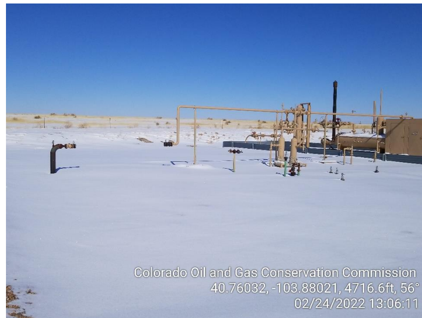
Photo 2 – Risers at Separators
