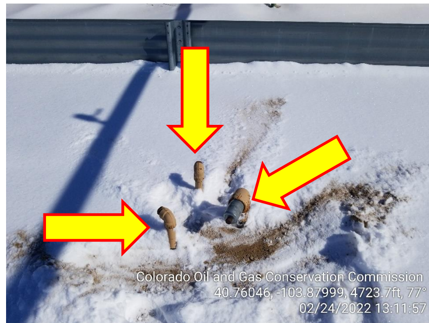
Photo 6 – Unmarked Riser
