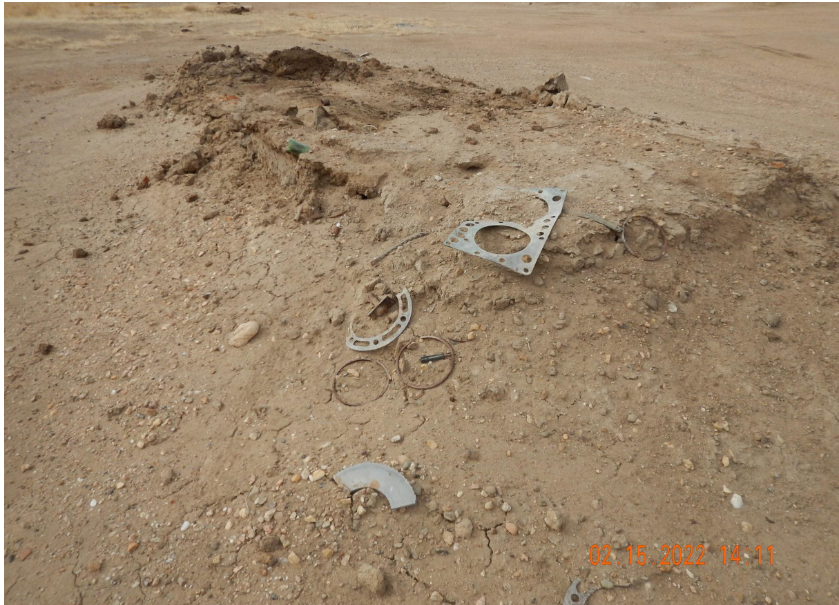
Photo 3. Photo taken from the wellhead. Photo illustrates Operator has not removed gravel and debris and recontoured the well location portion of the location.
