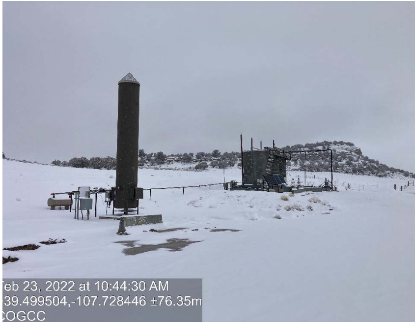
Location/ tank battery lacking battery signage
