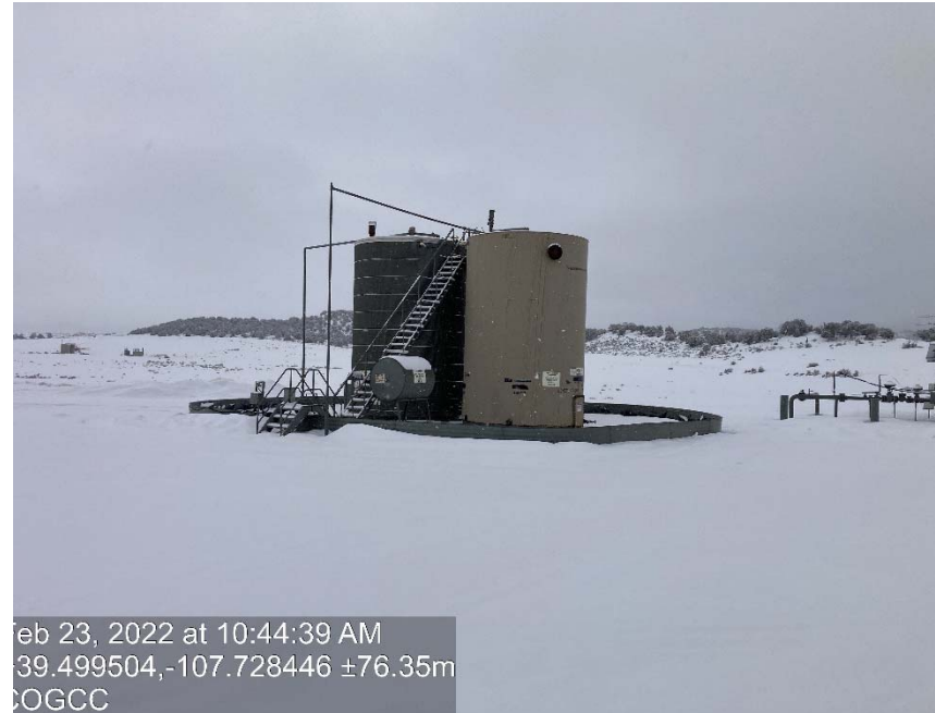
location/ tank battery lacking battery signage
