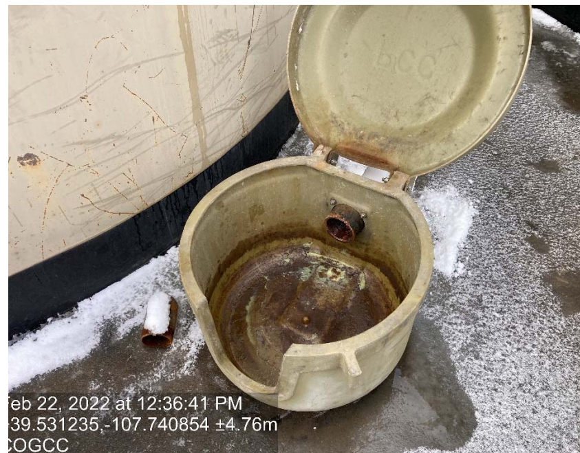
Missing plug/cap
