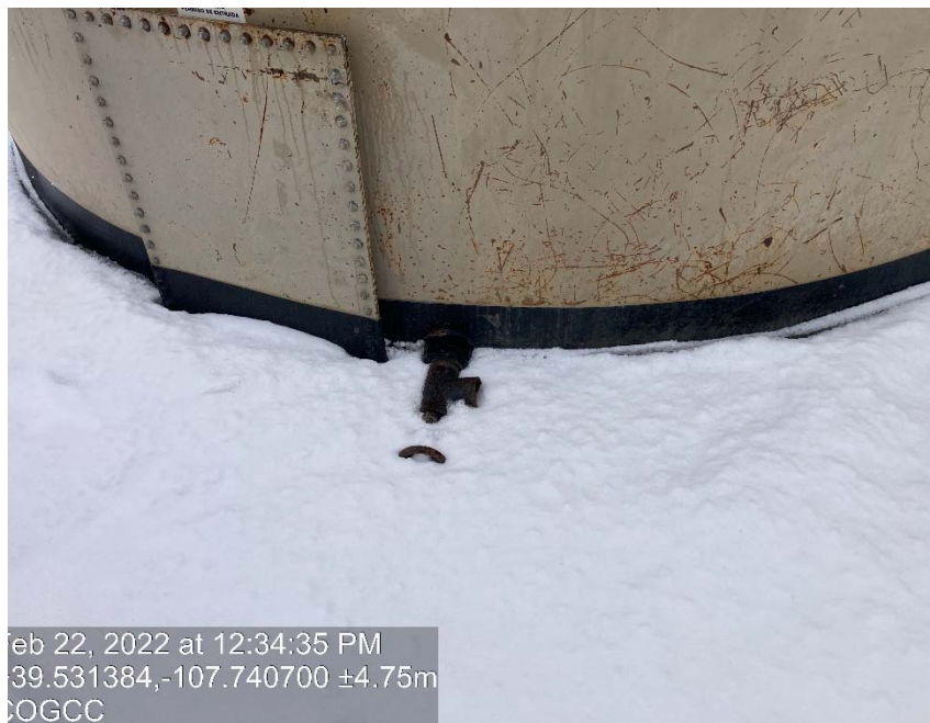
Missing plug/cap
