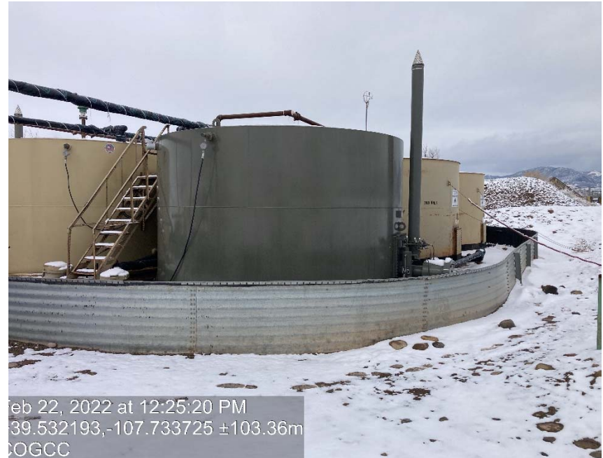
Tank not labeled or tied down
