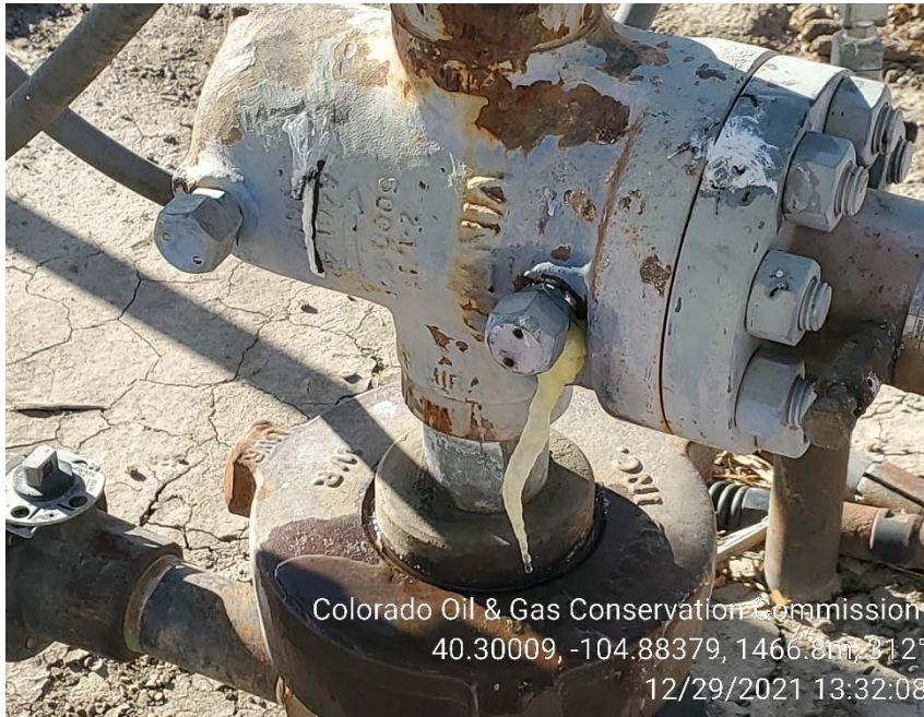
Master valve leak on 12/29/2022
