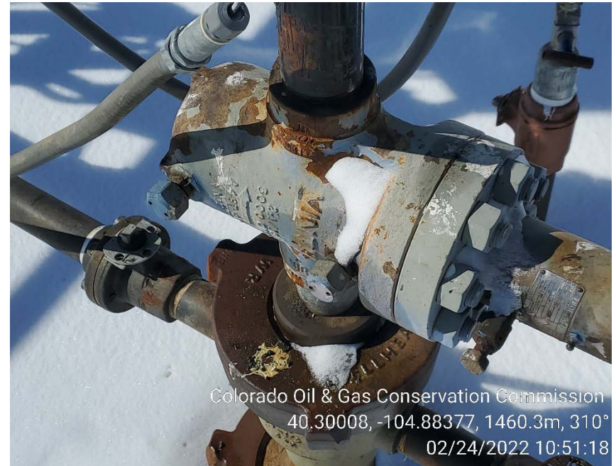
Master valve leak on 2/24/2022
