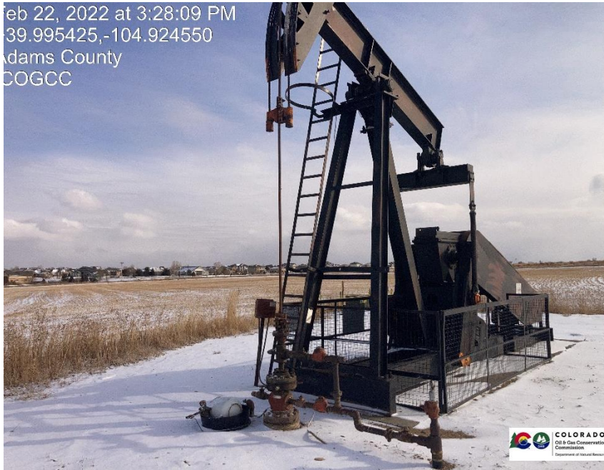
Pic 1 wellhead, electric equipment, pump jack
