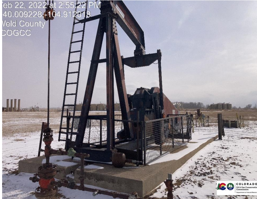
Pic 1 wellhead pump jack electric equipment.
