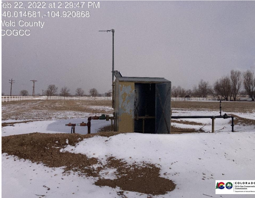
Pic 3 gas meter run
