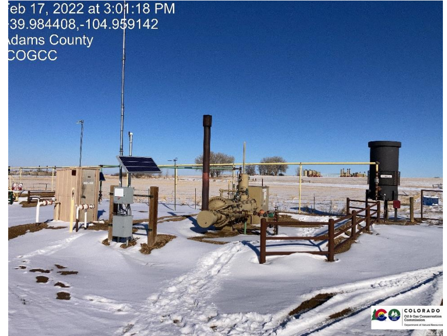
Pic 2 Gas meter run, Separator, ECD
