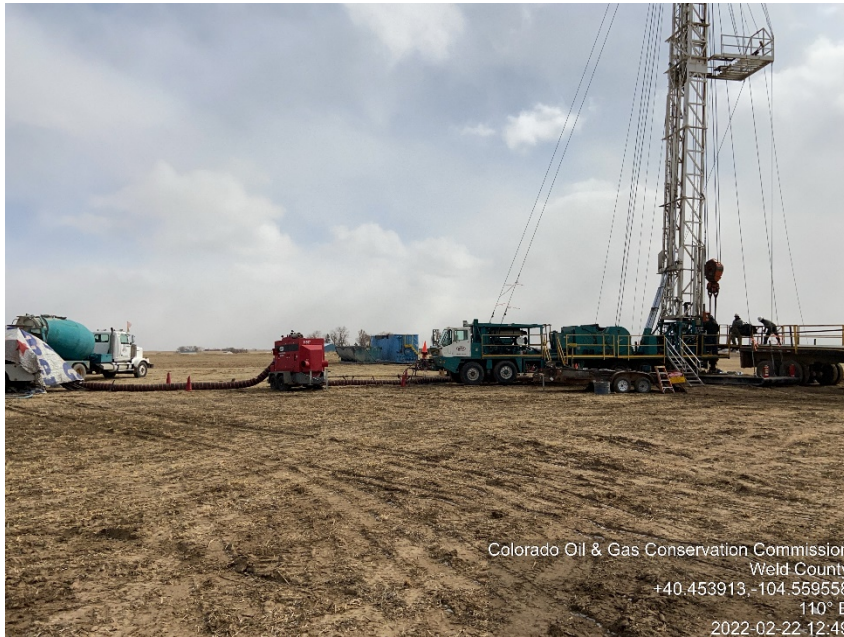
Photo #1 Rohr A 28-25 (05-123-32718) Wellsite Plugged & Abandoned | PA Plugging Operations: Cementing | WK Initial plugs cementing
