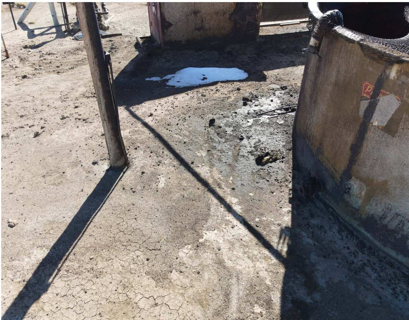
Spill from produced water and oil tank.
