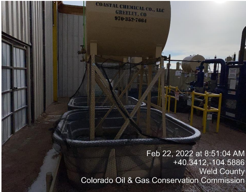
Photo #2 Bird Protector installed
