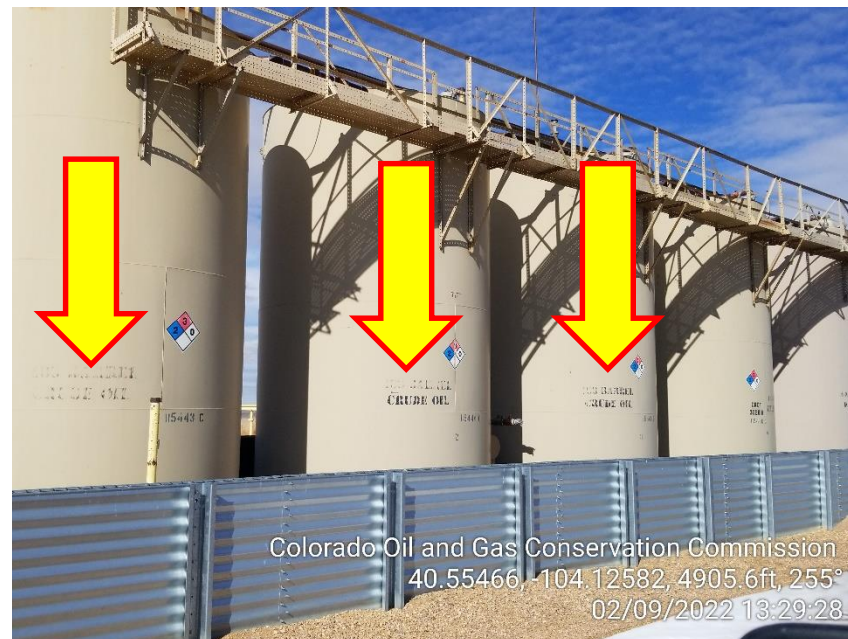
Photo 2 – Tank Battery – Content and Capacity Labels
