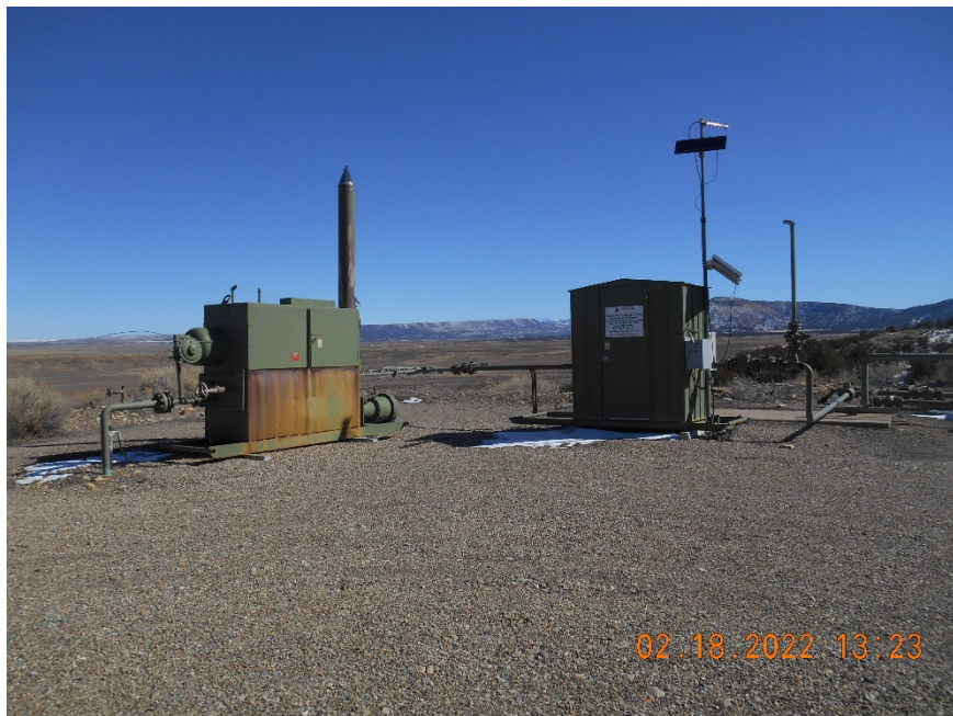
Separator and Meter housing
