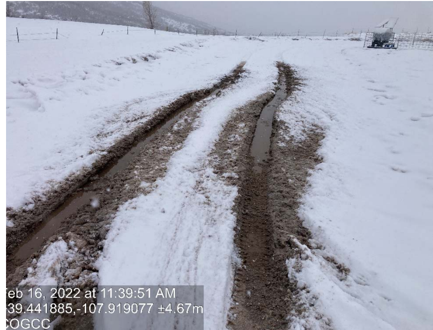
Lack of stabilization/compaction
