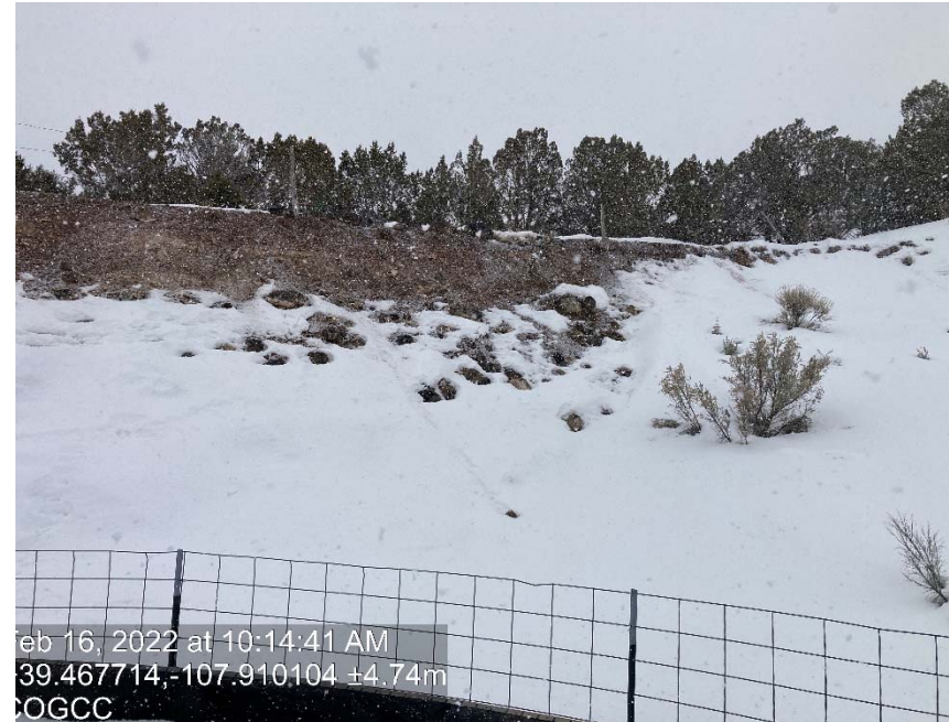
Cut slope still shows signs of lack of stabilization
