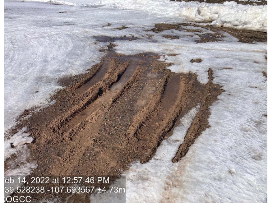
Lack of stabilization/compaction
