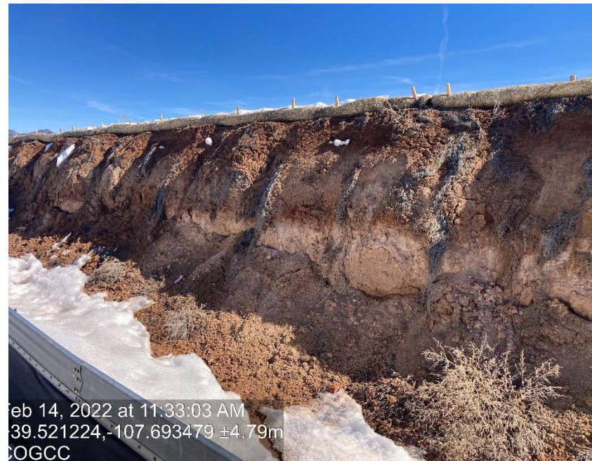
Cut slope not stabilized
