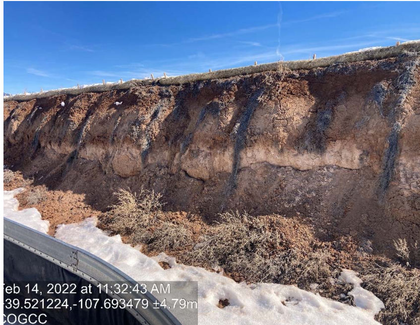
Cut slope not stabilized
