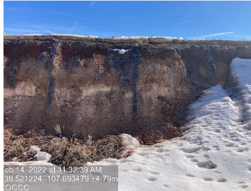
Cut slope not stabilized
