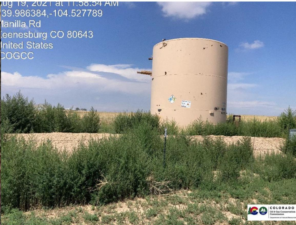
Here the Crude Oil Tank is situated higher than Produced Water Tank. They are both connected to the manifold in the Separator. A failed valve in the manifold could cause a gravity flow until the tanks equalize. The wells may also still be connected and could be the source of the overtopping. Easy access from Manilla Road and 160<sup>th</sup> Ave. suggests possible tampering.
