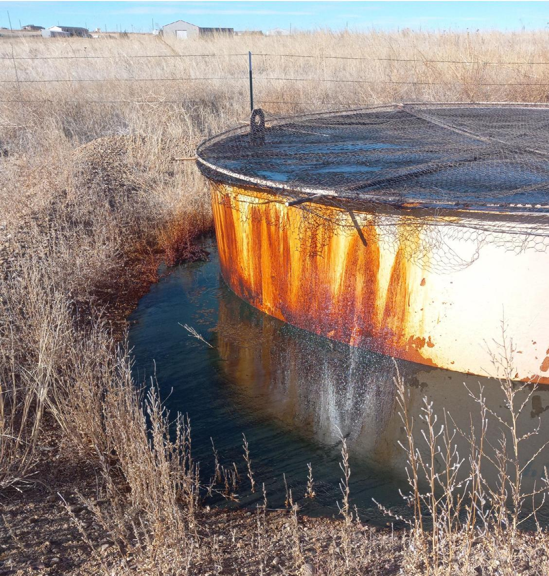
The overtopping on the produced water tank is encroaching on the secondary containment freeboard, but no longer appears to be flowing.
