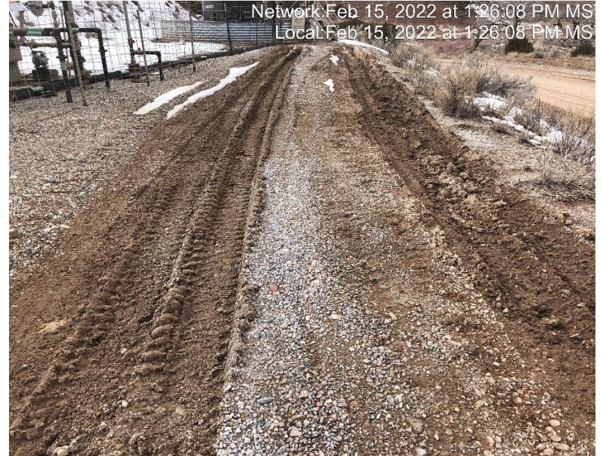
Photo #5969 Insufficient tracking controls at entrance to location.
