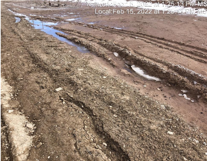
Photo #5967 Location lacks stabilization.
