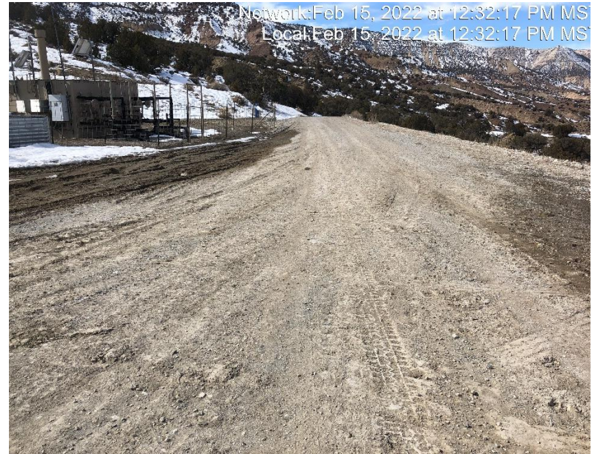
Photo #5964 Insufficient tracking controls.
