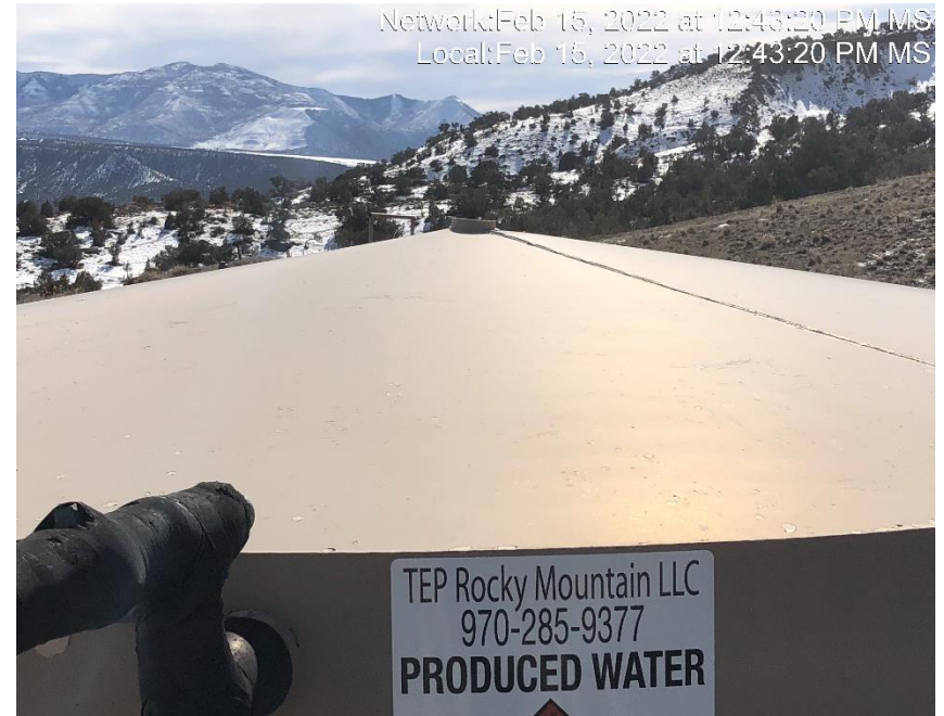
Photo #5965 Vent pipe on tank open ended.
