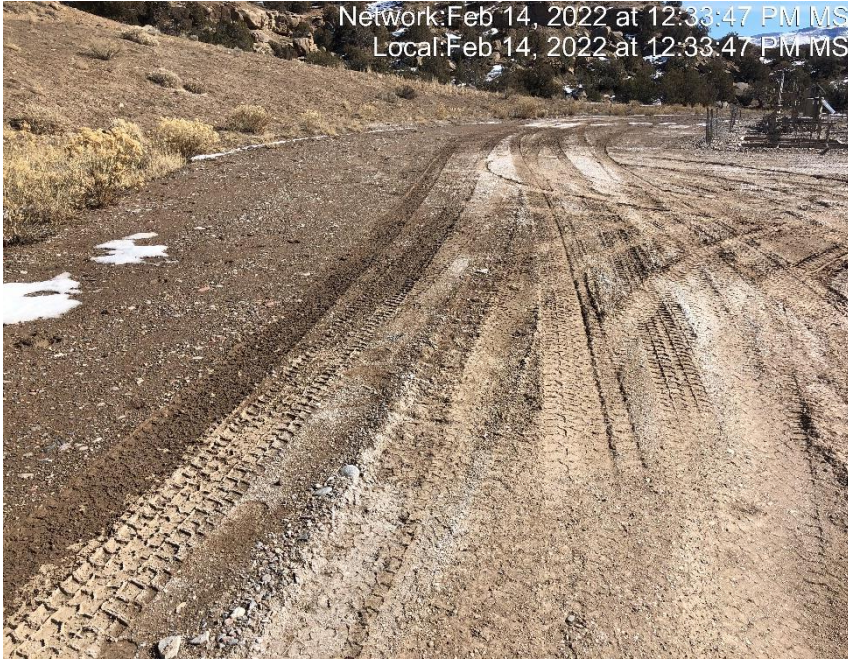
Photo #5955 Location lacks stabilization.
