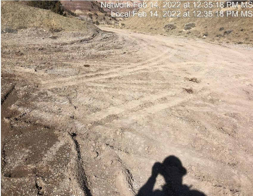
Photo #5957 Insufficient tracking BMP at entrance to location.
