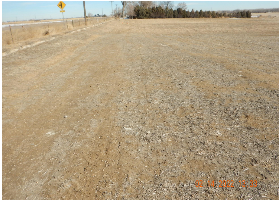
Photo 1. Photo taken from the associated offsite tank battery, facing East. Photo illustrates Operator has performed final reclamation activities with the evidence of drill rows.
