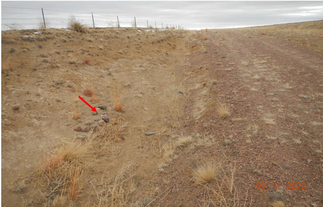
Photo 3. There is a rock check dam at this point which needs to be repaired.
