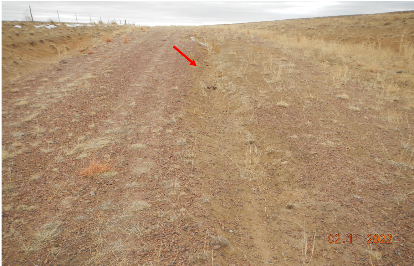
Photo 2. There is an erosion channel long the road at LatLong:38.74925,-104.55225. This area needs to be repaired and stabilized.
