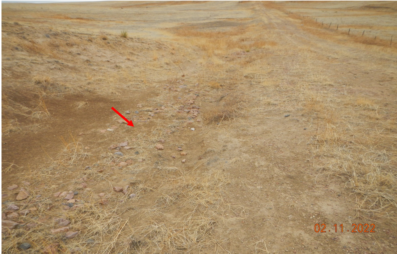
Photo 4. There is a rock check dam at this point which needs to be repaired.
