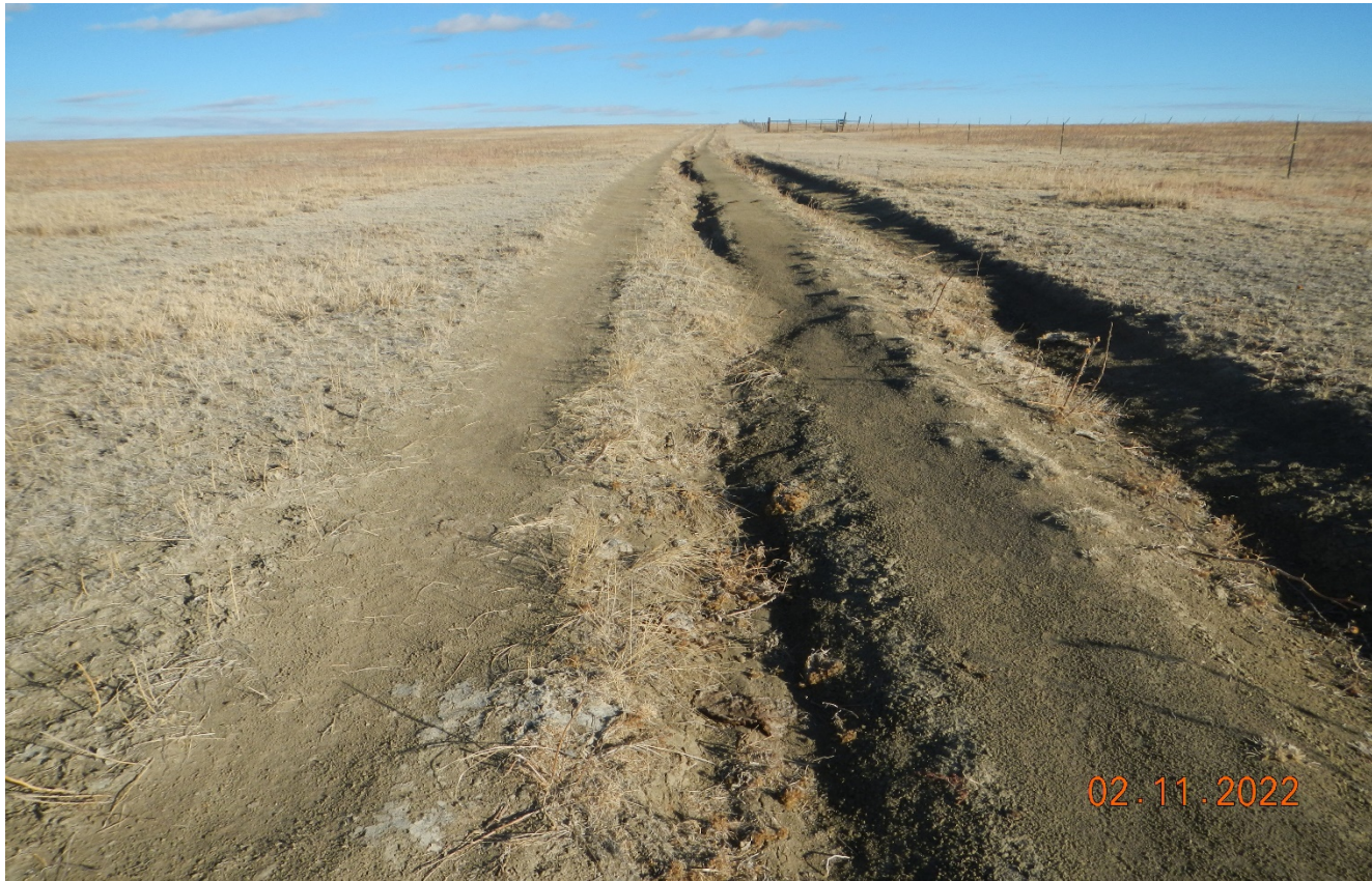
Photo 1. Facing north along the pre-existing access road. This area of erosion along the road needs to be repaired and stabilized. Approx. Lat/Long:39.19304,-103.54694
