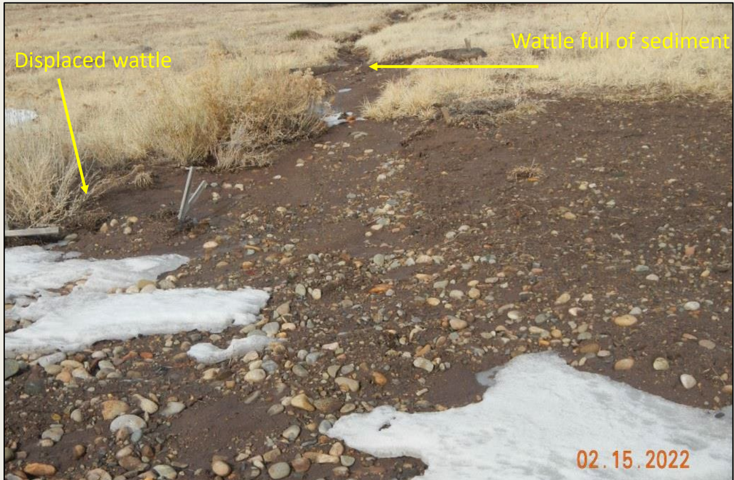
Photo 3. View of stormwater BMPs in the northern project area that need maintenance.
