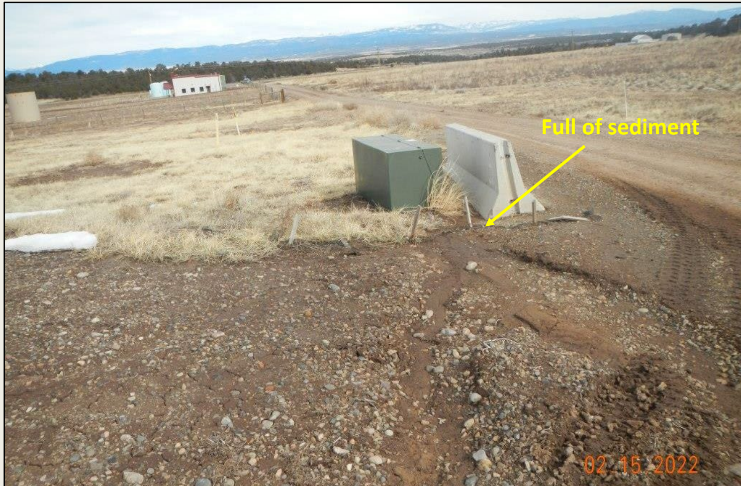
Photo 4. View of wattle at the well pad entrance that is full of sediment and is not an adequate BMP for this location. Maintenance is needed.
