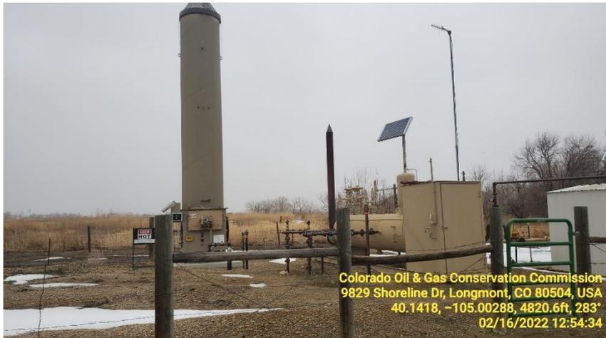
**Photo 9 ECD and Horiz. Heated Separator**
